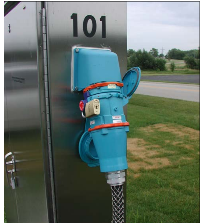
Unlike pin and sleeve devices, MELTRIC Switch-Rated devices can be padlocked in the on or off position to eliminate the dangers of tampering.
