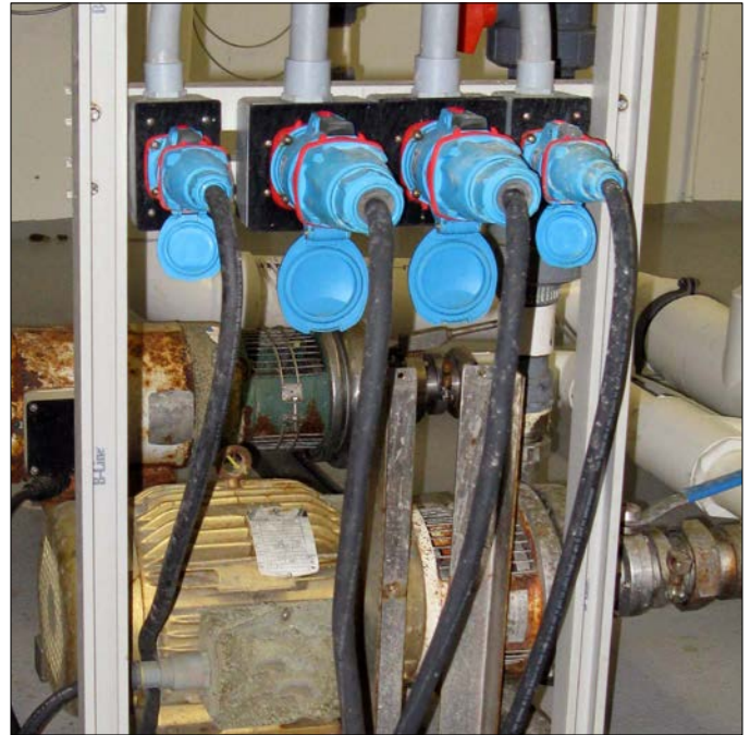
Four MELTRIC Switch-Rated connectors provide power to individual pumps used to empty holding tanks for various sizes of pickles.
