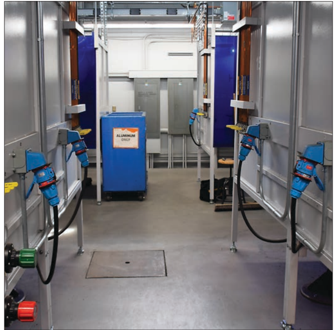
MELTRIC Switch-Rated plugs and receptacles provide power to 60 different welding workstations throughout the welding lab,
