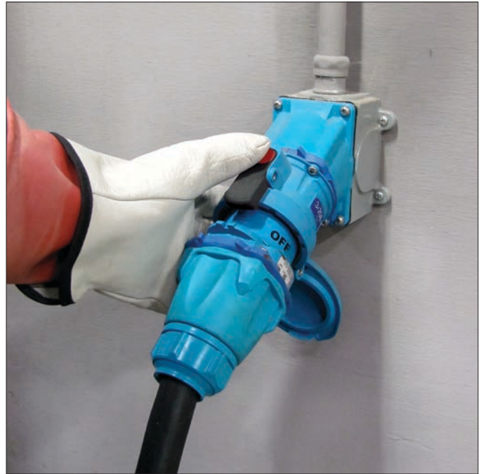
MELTRIC Switch-Rated plugs and receptacles meet NEC requirements as a 'line of sight' disconnect switch. Depressing the pawl on the receptacle (red dot) breaks the connection and ensures safe removal of the plug from the receptacle.
