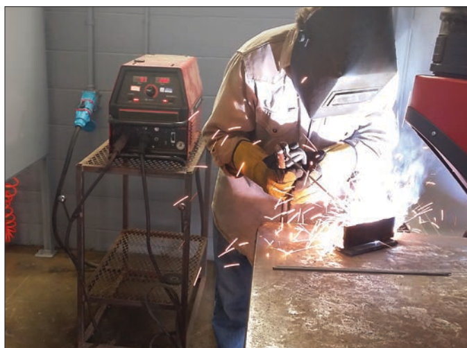
Changing out welding equipment in Odessa College's welding booths is easier with MELTRIC Switch-Rated plugs and receptacles. They feature an integral switching mechanism that allows safe make and break, even under full load.
