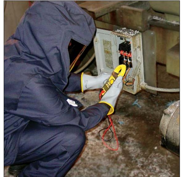
After opening the disconnect switch, a worker still needs to verify deenergization. Exposure to live parts is inevitable, so PPE is required.
