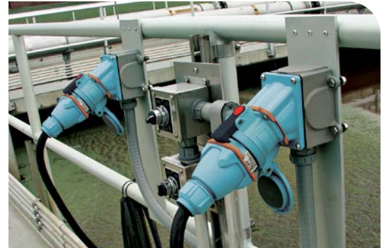
Electrical connections to submersible pumps for effluent water. Using a DECONTACTOR™ instead of a hardwired connection improved pump maintenance efficiency.
