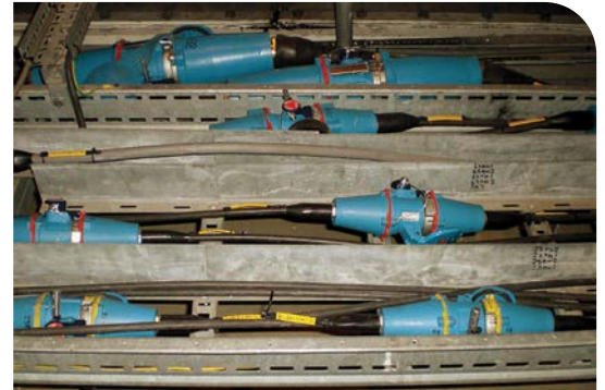
Switch-rated plugs and connectors allow technicians to safely disconnect and reconnect roof area power cables – simplifying turbine maintenance.
