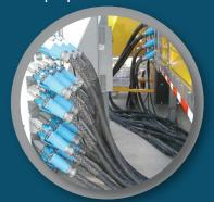
Incorporating Switch-Rated connectors into power distribution ensures that users can safely make and break connections.
