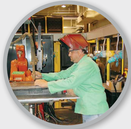
Switch-Rated plugs and receptacles eliminate the need for auxiliary disconnect switches at the ground level, saving space and connection time.
