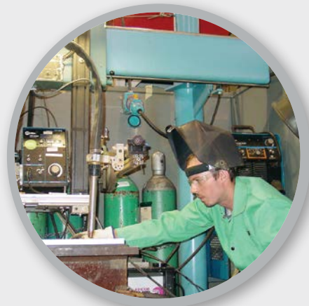
Switch-Rated plug and receptacle (background) enables technician to safely deenergize and relocate welding equipment.
