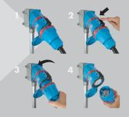
Press the button to quickly deenergize equipment; twist and remove plug.
