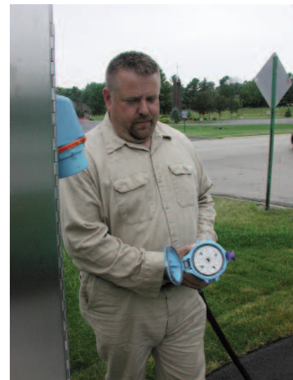
Connecting a generator to the lift station is fast, safe and easy, and an electrician is not required at the jobsite. When disconnected, the plug’s dead-front construction keeps workers safe by preventing accidental contact with live parts.
