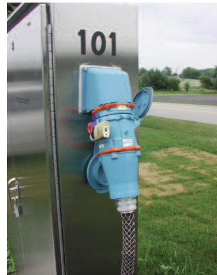
Unlike pin and sleeve devices, the Deconnector can be padlocked easily in the on or off position to eliminate the dangers of tampering.
