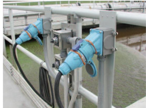
Closeup shows Meltric Decontactors for two adjacent mixers. Pressing the pawl on top of the device disconnects the power safely before the plug and receptacle can be separated.
