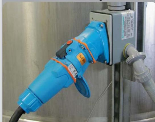
It is best to install the receptacle so it is pointing down with the plug pointing up. For washdown environments, a Threaded Handle with cord grip would have been a better accessory choice over the Nylon Handle shown.
