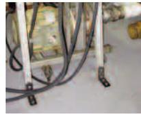
*Four Decontactors provide power to individual pumps used to empty the holding tanks that hold four separate sizes of pickles.*
