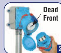
The plug and the receptacle can then be separated. The safety shutter prevents access to live parts.
