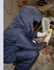
*After throwing the disconnect switch, a worker still needs to verify deenergization. Exposure to live parts is inevitable, so PPE is required.*
