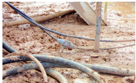
Adverse conditions include water, mud and temperature extremes, yet the Deconnectors have continued to operate reliably since being installed.
