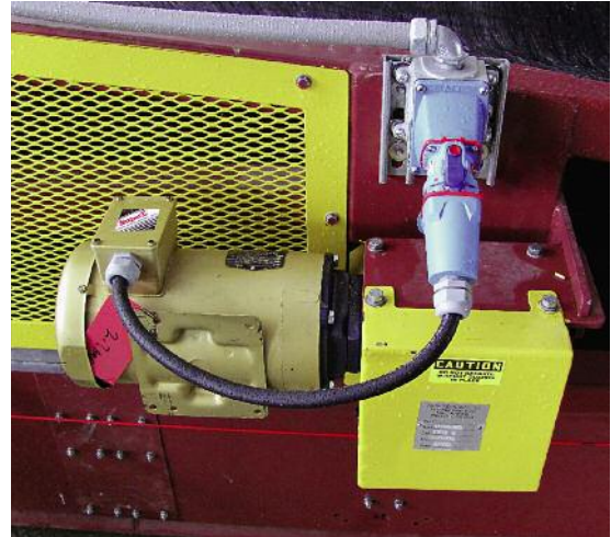
Installing a Meltric Decontactor Series switch-rated plug/receptacle between a motor connection box and the power line feed eliminates all hardwiring tasks during motor changeouts. Load breaking is performed in seconds by pushing the red, spring-loaded, pushbutton pawl on the plug's casing.
