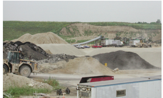
Portable conveyors and crushers at this Payne & Dolan aggregate operation are easier to move as they follow the material source because Meltric plugs and receptacles simplify power connections.
