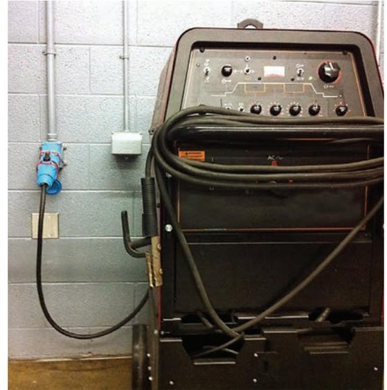
*Exclusive safety features make Meltric's Switch-Rated plugs and receptacles ideal for connecting power to welding machines at Odessa College.*
