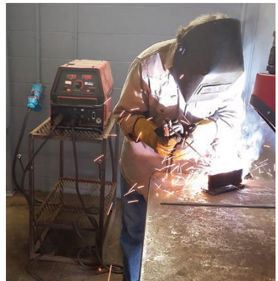
Changing out welding equipment in Odessa College's welding booths is made easier with Meltric Decontactor switch-rated plugs/receptacles since they feature an integral switching mechanism that allows safe make and break even in overload conditions.
