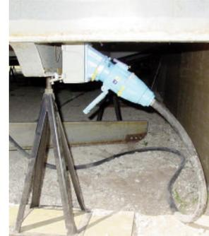
*A male inlet is installed at the mobile classroom corner opposite the panel. The female connector is easily mated to the inlet providing a safe and neat power connection.*
