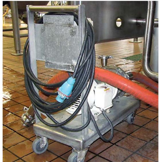
*At Bell's Brewery, portable pump carts are connected with Meltric DecontactoRs which combine the safety and functionality of a disconnect switch with the convenience of a plug and receptacle. Their integral switching mechanism allows users to safely make and break connections under full load and provide significant protection in overload and short circuit conditions.*
