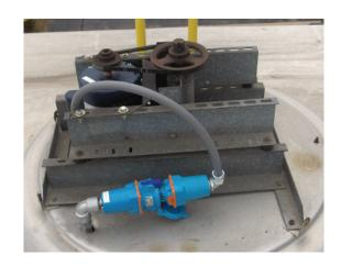
"With the Meltric connector installed there is no need to physically mount a disconnect within sight for smaller
