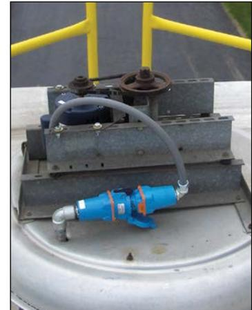
"With the MELTRIC connector installed there is no need to physically mount a disconnect within sight for smaller motors on the roof so this is a good solution for us" said Monique Newell, a maintenance specialist at Scientific Protein Laboratories (SPL)
