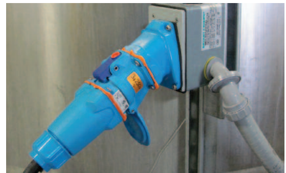
Meltric's Decontactor plugs and receptacles are an approved 'line of sight' disconnect. Pressing the pawl on the receptacle (red dot) breaks the load and ensures that the plug can be safely removed.
