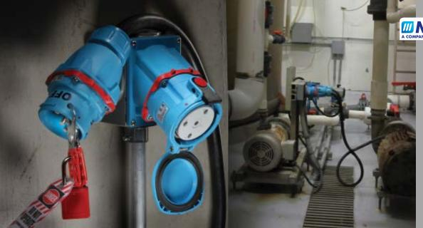
NELIRIC Switch-Rate lugs & receptacles an be easily locked ut and tagged out, nly your lock and an are needed
