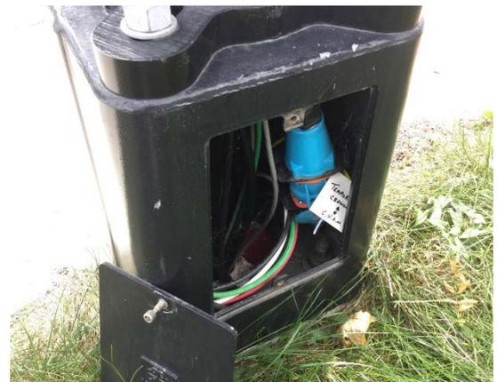
*A special box was built by Trelec to install the DSN60. This box goes between the concrete base and the pole.*
