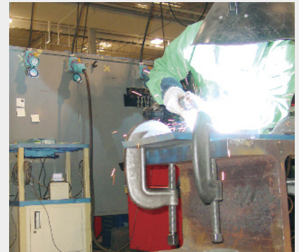
Switch rated welding receptacles (background) are connected to overhead busway system via cord drops.
