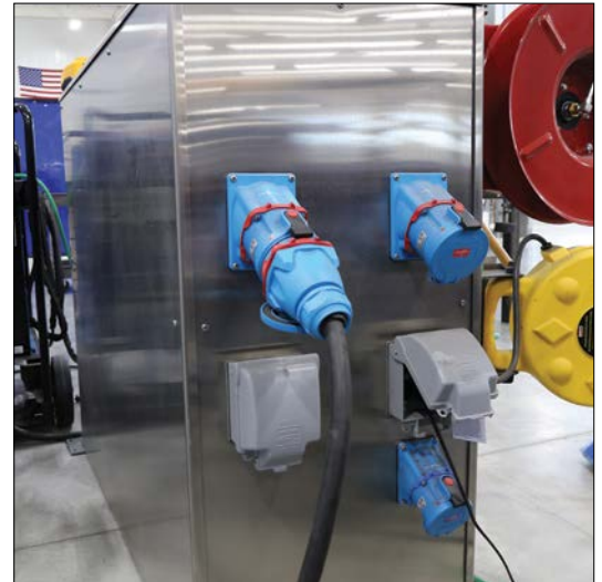
MELTRIC Switch-Rated plugs and receptacles combine the safety and functionality of a disconnect switch with the convenience of a plug and receptacle in one device.
