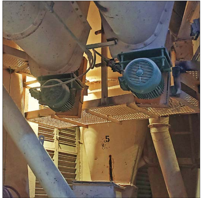
With the DXNs' direct motor mounts, Purina Mills saved more than $75,000 on electrical boxes and wiring costs. MELTRIC DXNs provide convenient mounting options, even in areas with limited space.
