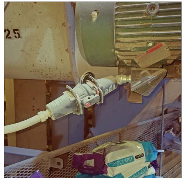
MELTRIC DXNs provide safe, reliable connections in Hazardous Locations where dust and gas are present. DXNs are rated for use in Div 2, Class I and II, Zones 1 and 2, 21 and 22.
