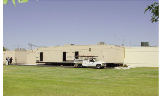
Mobile classroom buildings such as this one being set up at Elaine Wynn Elementary School are easier to move since the Clark County, Nevada School system started using Meltric switch-rated plugs and receptacles instead of hard wiring electrical power
