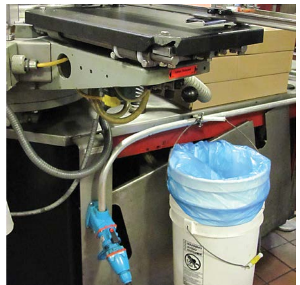
MELTRIC Switch-Rated connectors meet NEC 'line of sight' disconnect requirements. Users can safely make and break electrical connections under full load.
